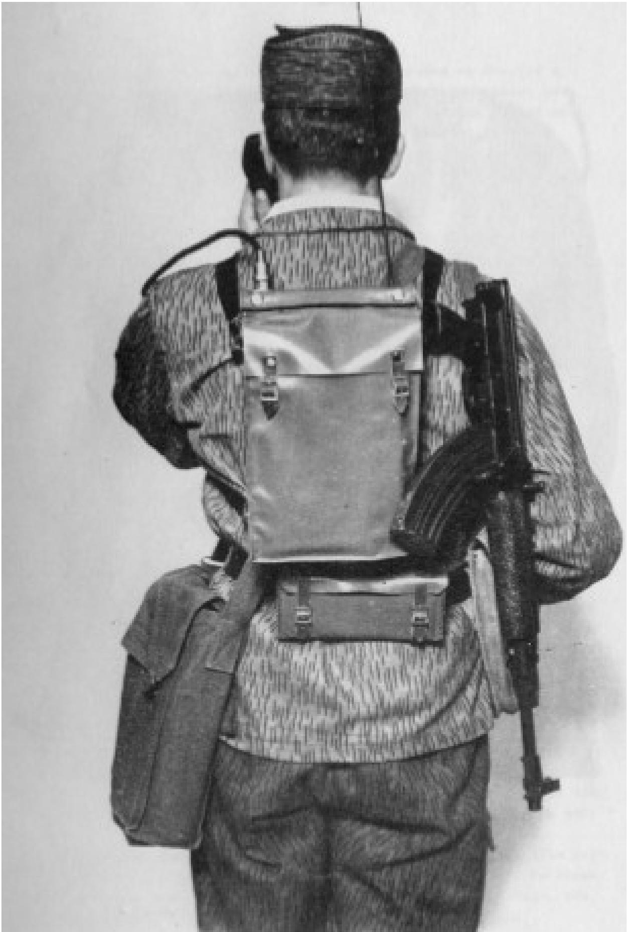
*Figure 9: The radio in a bag worn on the back – rear view – spare battery bag horizontal*
